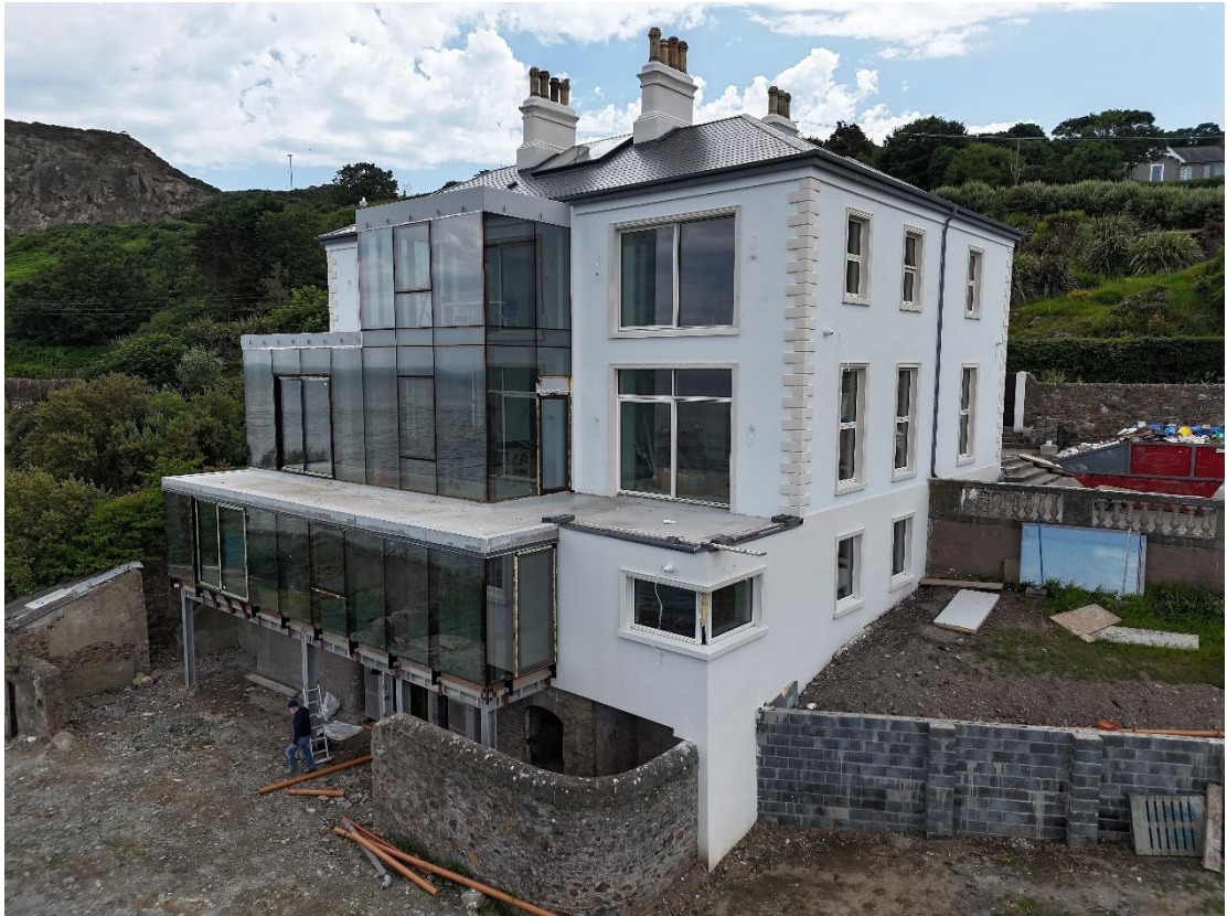
Figure 1. Current condition of the site
