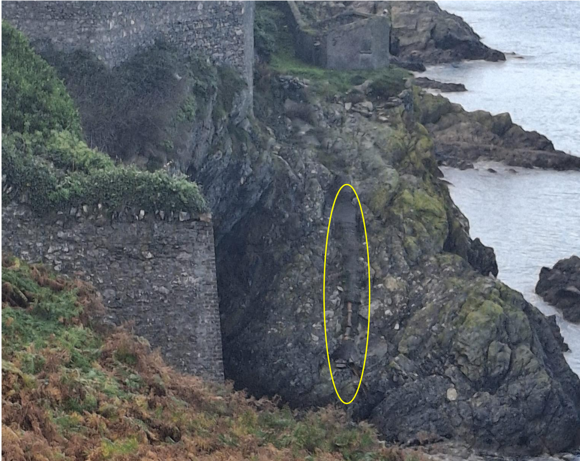
Figure 5. Cliff face outfall (Clay pipes within yellow outline)
